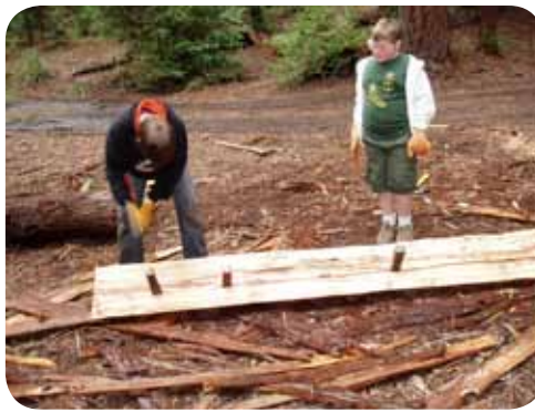
Work party attendees helping to split wood to make new spars for the fence around the redwood grove.
